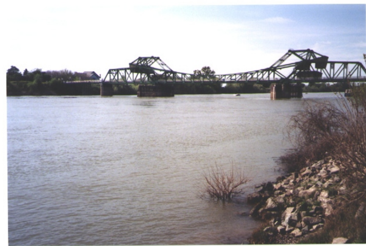
Sacramento River at Freepoint
