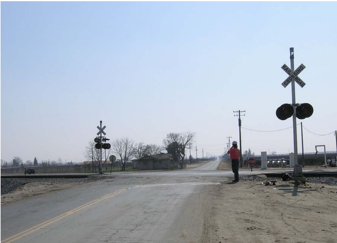
Figure 8: Grade crossing at Poplar Avenue looking south. The (five) embedded lights under test run across the width of the road parallel to the white limit (double) line and just north (foreground) of it. Other than being too far to the right, the perspective of this photograph is approximately that of a driver approaching the grade crossing.
