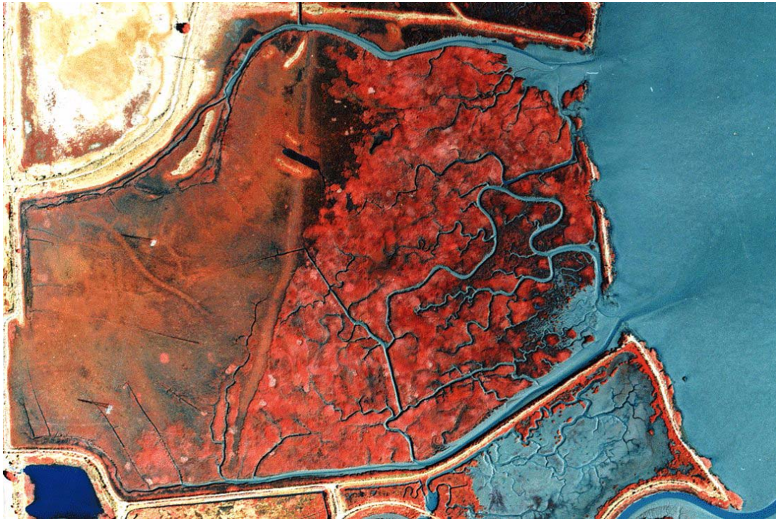
Figure 7 Aerial photograph showing erosion of the outer levee at Muzzi Marsh 22 years after restoration (1998 photograph)
