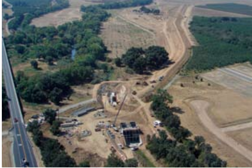
Setback levee being constructed near Bear River
