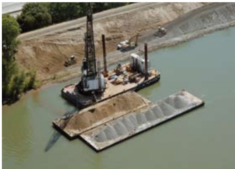
Levee repair site on Sacramento River
