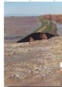
Levee Break - Flood of '97
